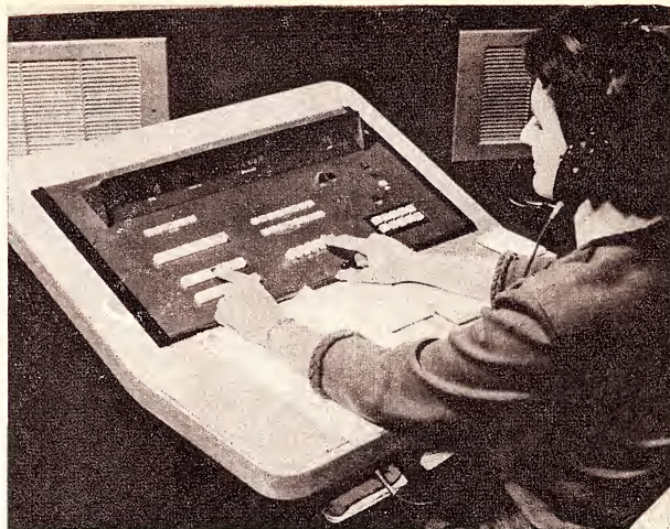
The operators' consoles have push-button controls, arranged to allow two-handed operation. The keys in the bottom row are those most commonly used.
