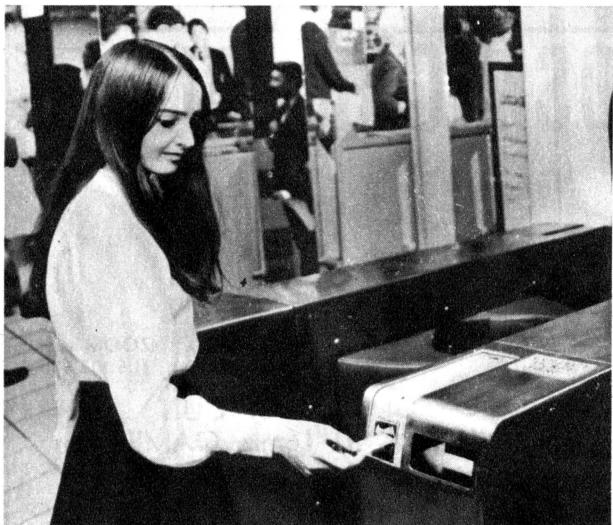
A visitor to a London exhibition tries one of the new electronic gates that operate throughout the Victoria Line, the new section of London's underground which opened recently. The automatic gates, operated by magnetically-encoded tickets, control passenger entry and exit at all stations. When completed, the 14-mile long "tube" with its 16 stations under the heart of London will have a peak capacity of some 25,000 passengers an hour in either direction.
