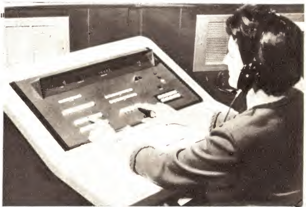
One of the operator's consoles of BP's electronic private telephone exchange.
