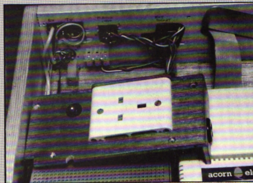
Internal wiring layout with the cover removed
