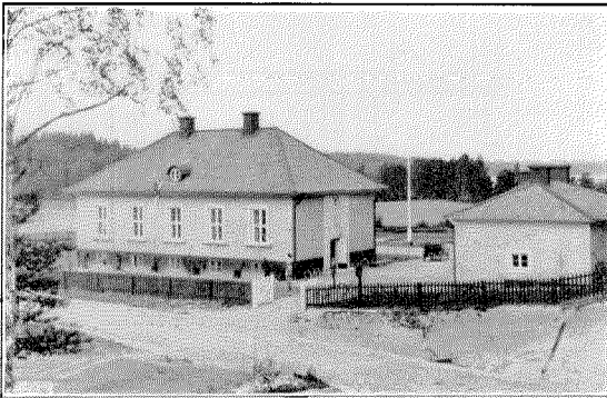
Figure 6—Repeater Station at Västerlång
