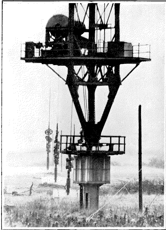
Figure 13—Base of Antenna Mast
