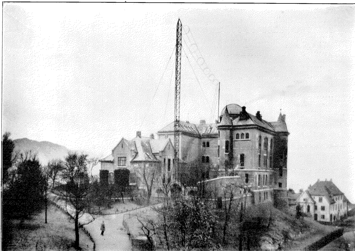
Bergen School of Navigation. The antenna is part of a Western Electric type radio broadcasting station furnished for temporary use pending completion by Standard Electric Aktieselskap, Oslo, of a permanent 1-kw. installation for the Bergen Broadcasting Company
