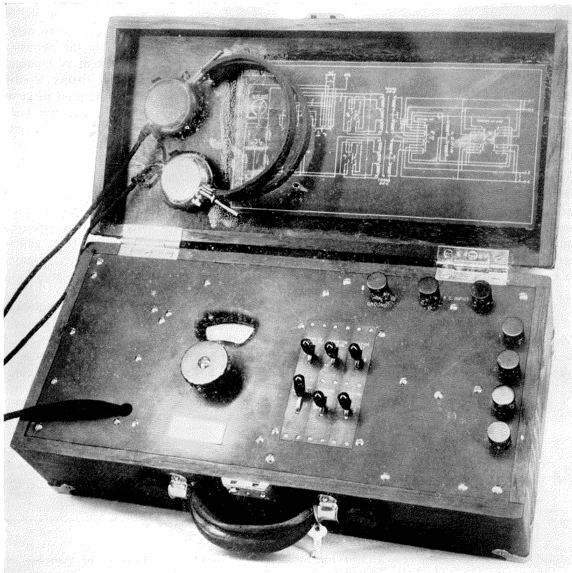
Figure 8—Crosstalk Measuring Set
