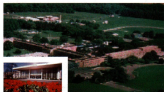
The David Saroff Research Center in Princeton, New Jersey, is one of the world's leading R&D facilities.
