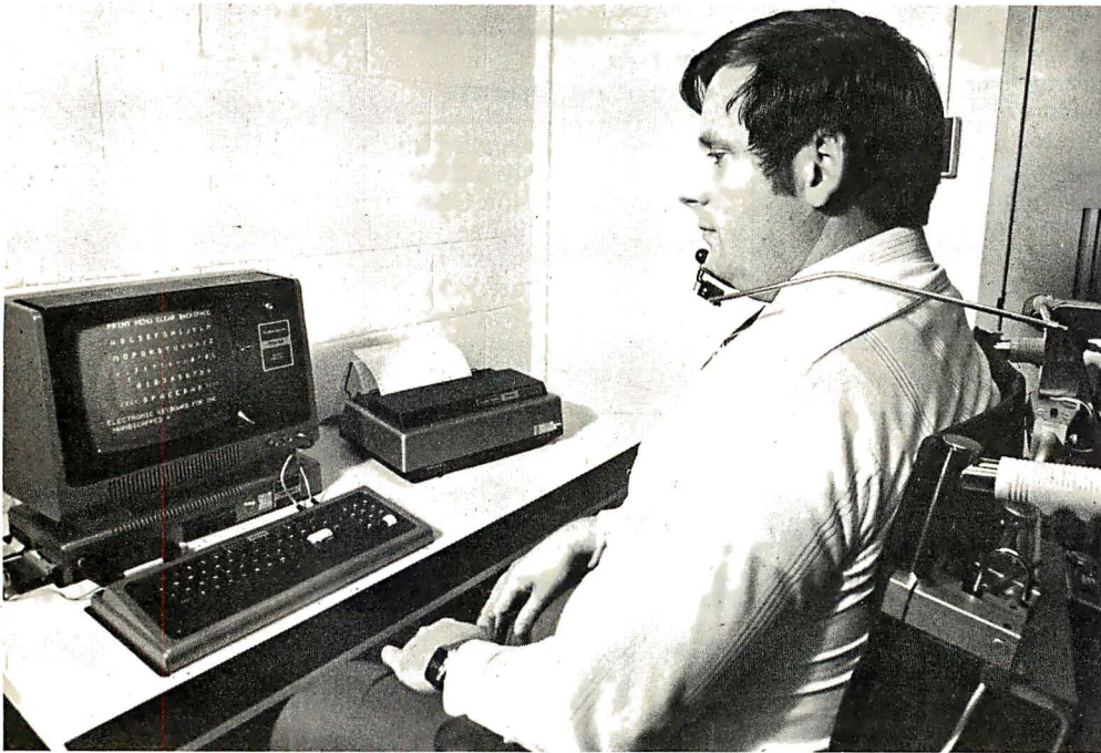
Photo 1: Personal computers can give the handicapped access to everyday activities. Here, a Johns Hopkins engineer demonstrates typing on a computer-aid electronic keyboard activated by a chin controller. The Johns Hopkins National Search for Applications of Personal Computing to Aid the Handicapped hopes to uncover similar applications.
