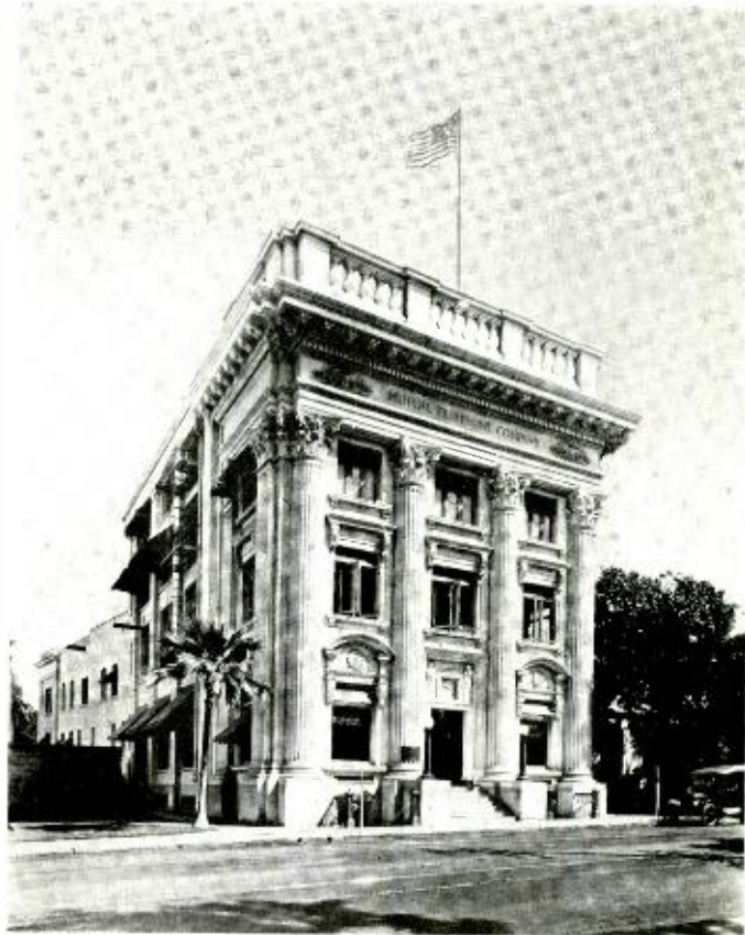
Main office building of the Mutual Telephone Company, Honolulu. This is a splendid example of the many modern buildings in Honolulu
