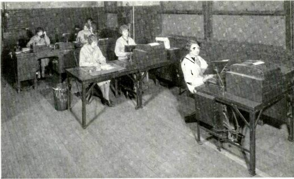
Printer equipment as it is today
