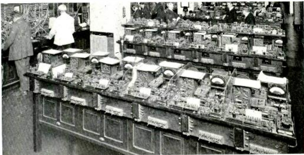
Fig. 1—Long-lines telegraph repeater test-board room showing the old-style apparatus
