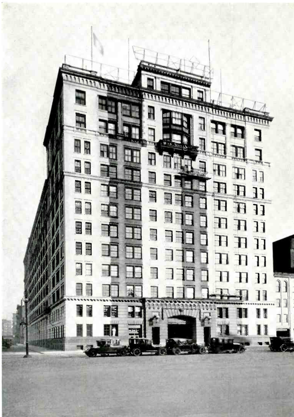
Our Building Has a Bath: To match the pristine freshness of the addition, the older part was cleaned— the brickwork chemically, the stone by sandblasting
