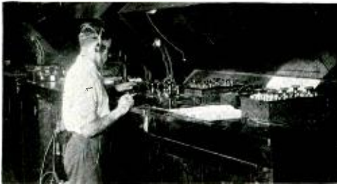
R. A. Chegwidden measures the constants of permalloy cable with an impedance bridge
