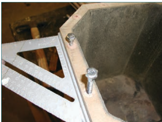
Photo 6: Pictured are dowel rods, glued into holes in which to thread lag screws
