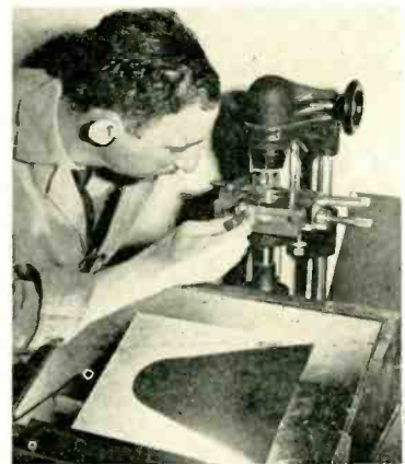
Fig. 3. Each diamond stylus must be inspected carefully on a shadowgraph.
