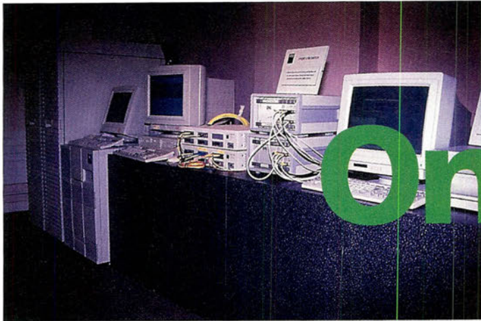
It's all controlled from here – at the back on the left is the ICL video server.
