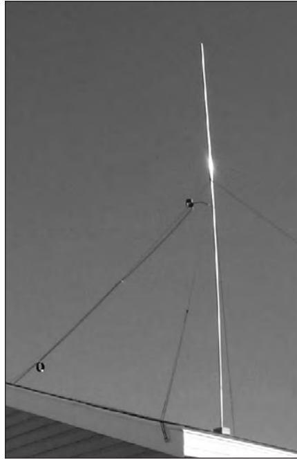
Fig 21.58 — The HVD installed at K8CH. An eye screw that is used for securing one of the guy lines is visible in the foreground. You can also see the two choke baluns that are used in the feed system (see text).
