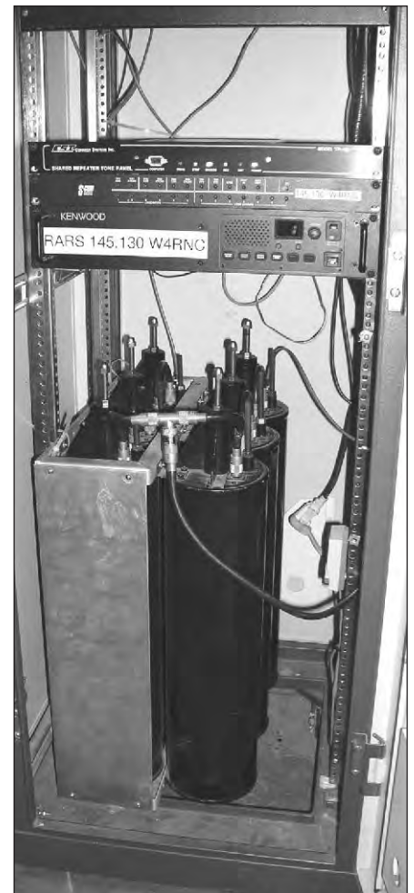
Fig 18.6 — The W4RNC 2 meter repeater includes the repeater receiver, transmitter and controller in the rack. The large object underneath is the duplexer. [Photo courtesy Gary Pearce, KN4AQ]
