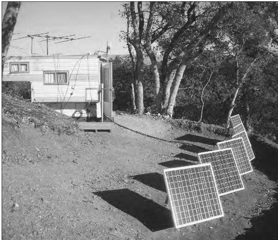
Fig 29.30 — Solar panels can be used to charge a bank of batteries to supply power. Effective off-grid power requires an accurate and conservative estimate of power needs and available energy sources. [Rick Hilding, K6VVA, photo]
