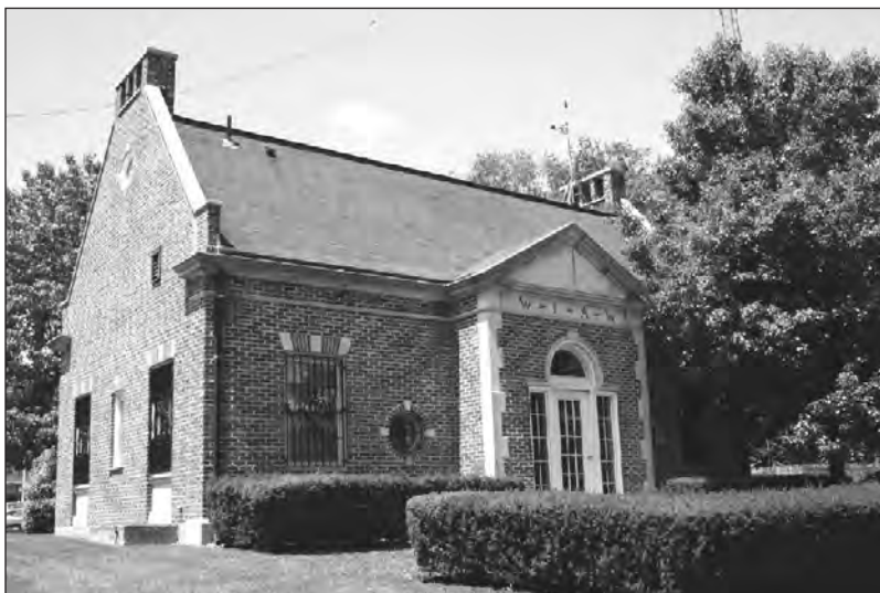
Fig 1.9 — This iconic brick building houses W1AW, the station operated by the ARRL in Newington, Connecticut, and known around the world. W1AW memorializes Hiram Percy Maxim, one of the founders of the ARRL. Visitors are welcome and often operate the station. [Rick Lindquist, WW1ME, photo]
