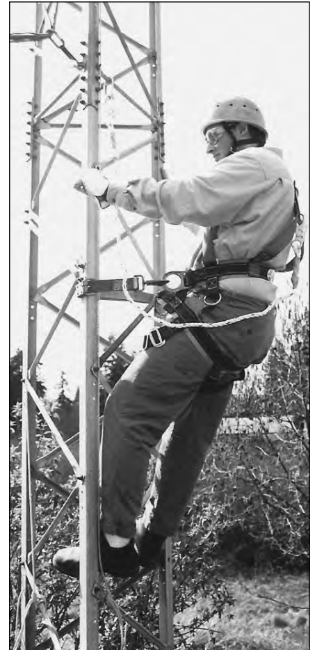
Fig 28.21 — The fall-arrest lanyard is above the climber so that the climber can climb up to it. The fall-arrest and positioning lanyards are then "leapfrogged" so that the climber remains attached to the tower 100 percent of the time. (K7LXC photos)
