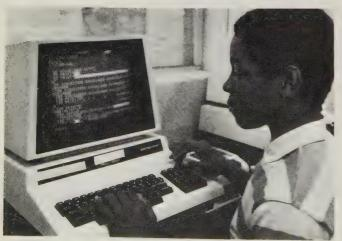
The keyboard is really just a set of switches. They are connected to the computer **processor**, not the screen. The screen, which is also connected to the processor, shows what you type only if the processor says to do so.
