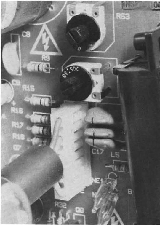
FIG. 6-17 This connector also carries a high voltage for the CRT. Again, don't touch.
