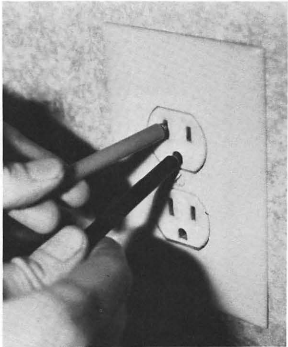
FIG. 6-3 Checking an outlet with a meter.
